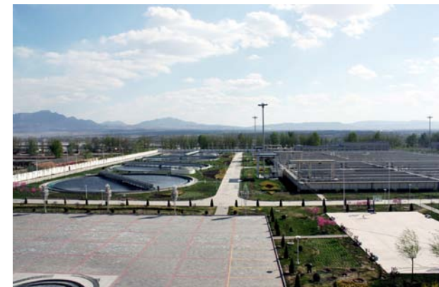
Xuanhua Wastewater treatment plant
