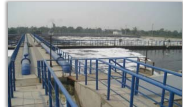
Tianjin WWTP, China
